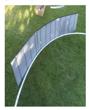
Step D: Join the upper frame segments to the wall panels.
